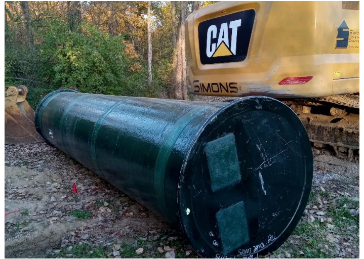
Above: Work on the lift station (now operational)
